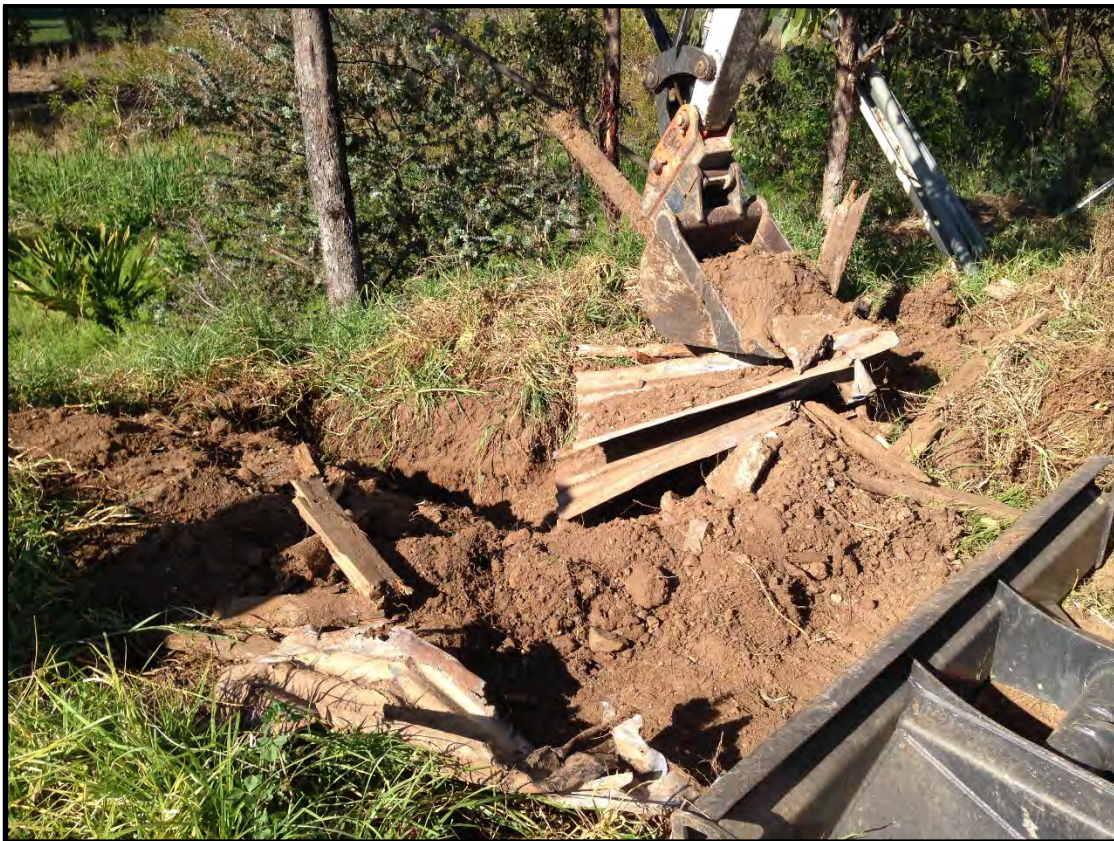
Photo 4: Facing southwest – Test pit 1 (TP1) example of waste types in the soil mounds.
